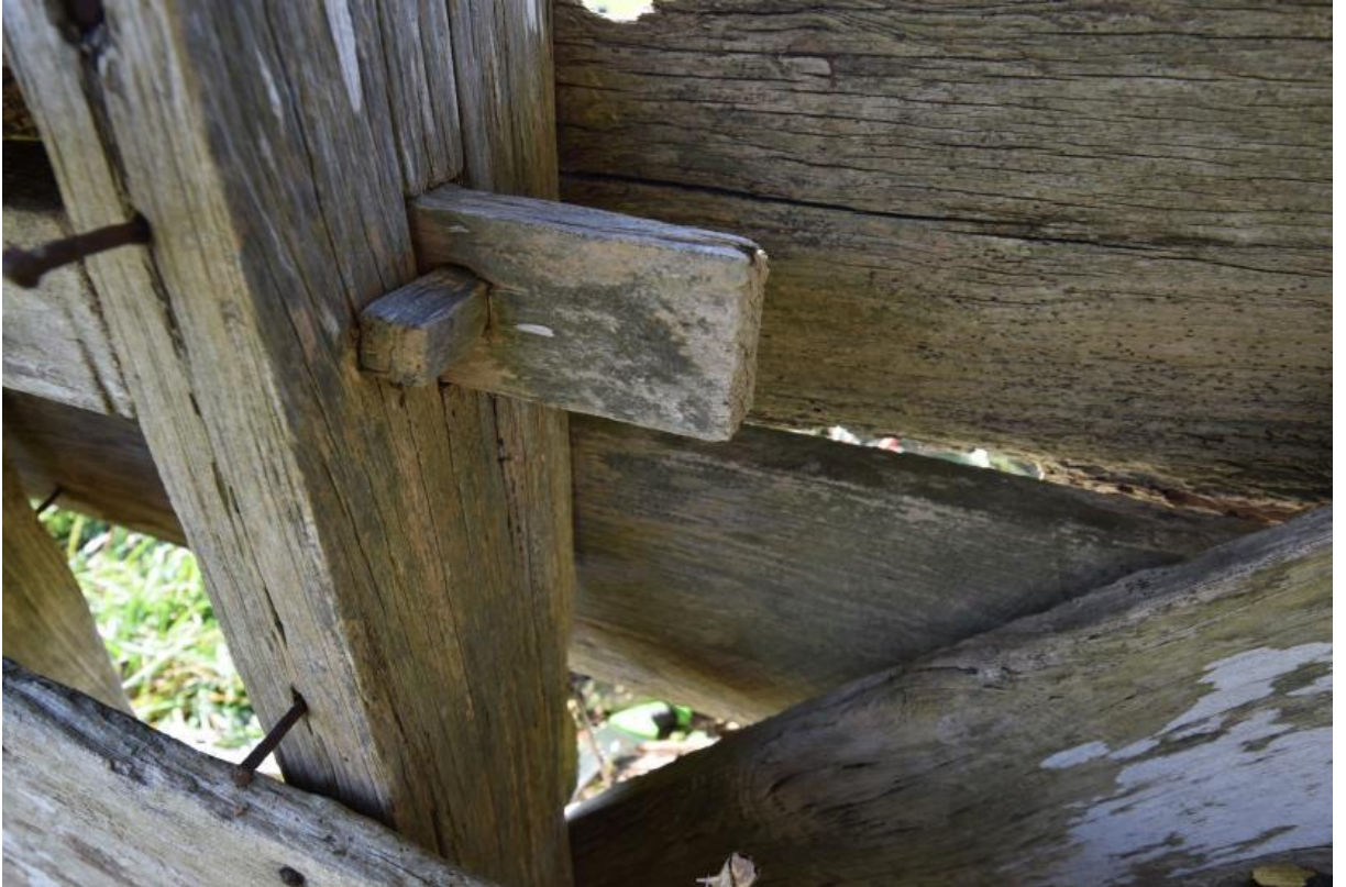
Figure 7. Example of mortise and tenon construction (joint with peg) and hand-made iron nails in the transit annex. Kerry Pollock, Heritage New Zealand Pouhere Taonga, 12 September 2019.
