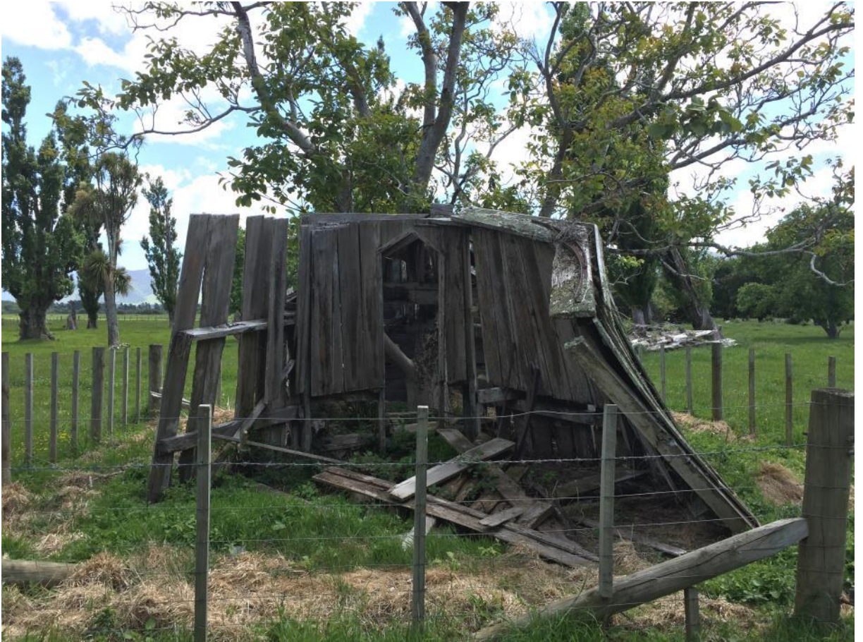
Figure 6. Interior of the equatorial room from the east. The apex-shaped door opening between the equatorial room and the transit annex is in the middle. Note the iron channel that remains fixed to the top (at right in the foreground). Christine Barnett, Heritage New Zealand Pouhere Taonga, 20 November 2019.
